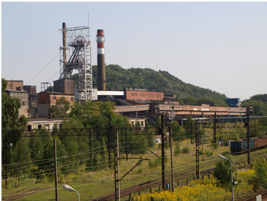
Debiensko Hard Coking Coal Project showing existing shafts and railway. Source: Company
